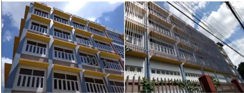
COMPLETION OF IT BUILDING (CONSTRUCTION OF 5-STOREY IT BUILDING PHASE VI) EXISTING CONDITION
