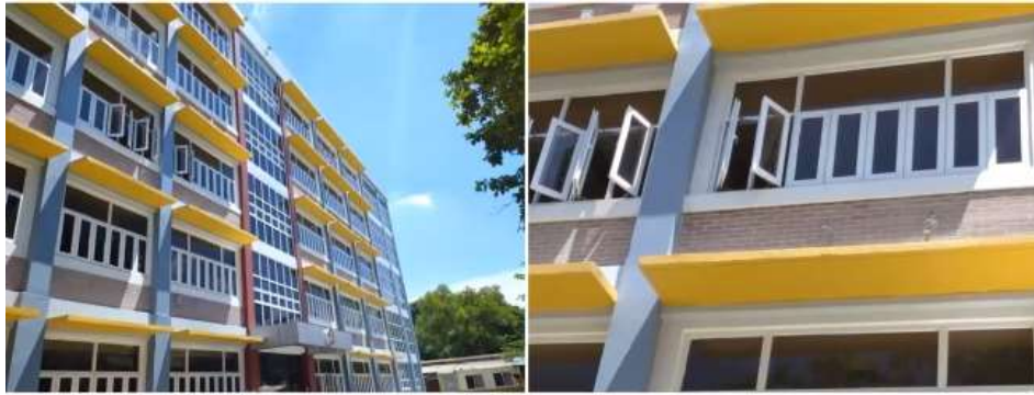
COMPLETION OF IT BUILDING (CONSTRUCTION OF 5-STORY IT BUILDING PHASE VI) EXISTING CONDITION
