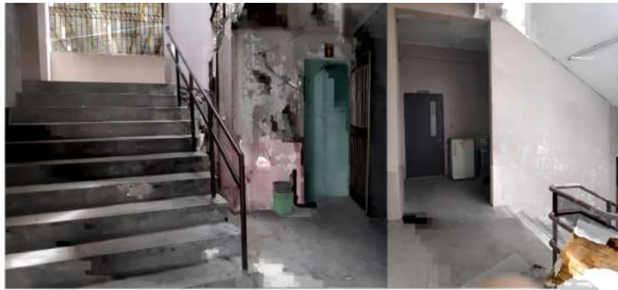
COMPLETION OF SCHOOL OF APPLIED ECONOMICS BUILDING EXISTING CONDITION
