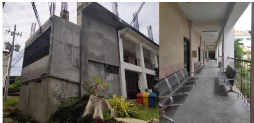
COMPLETION OF SCHOOL OF APPLIED ECONOMICS BUILDING EXISTING CONDITION
