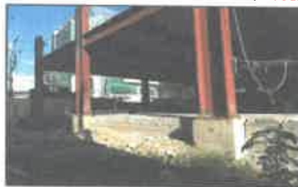
10 Pre-bid Conference 2018-29/Infra (COE Laboratory En'g Bldg Phase 2)
